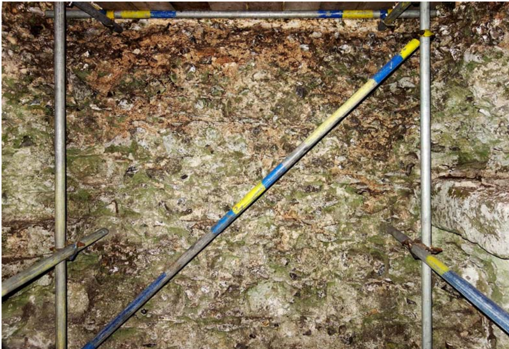
Figure 19. North internal wall face of eastern half of gatehouse at ground level showing banding of corework.
