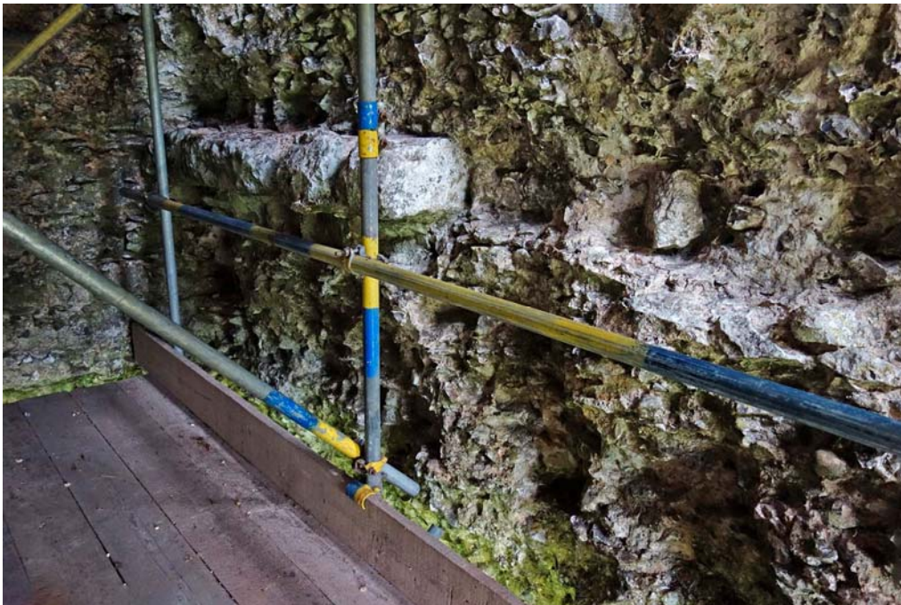
Figure 20. Blocks on inner face of east wall of gatehouse, identified as remains of the floor of the first-floor room.
