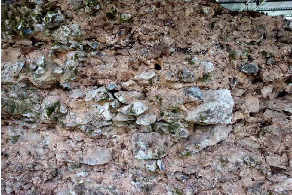
Figure 28. North wall of eastern first floor chamber. Banding of corework.
