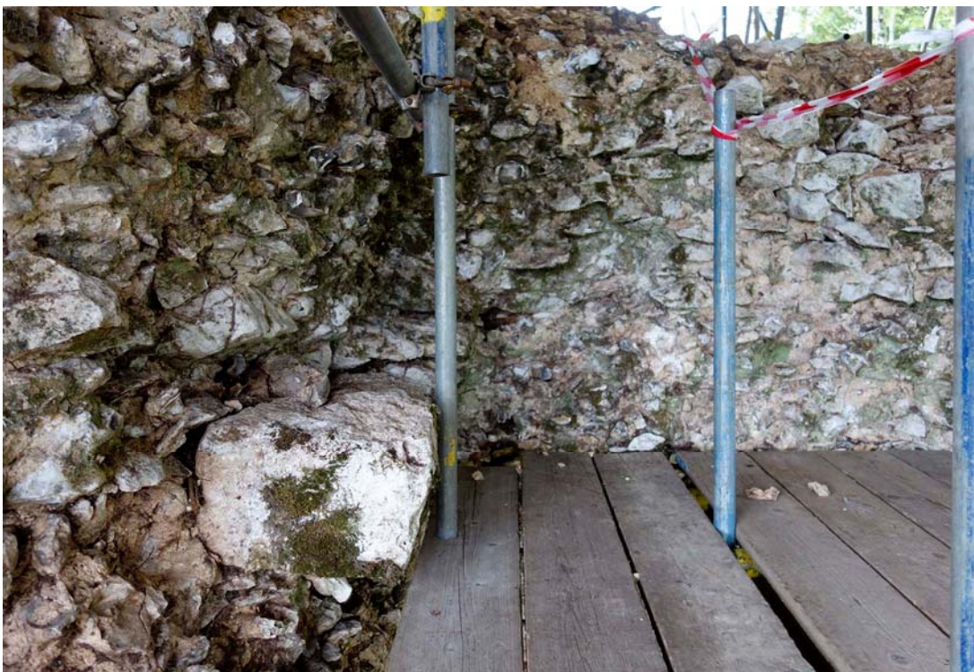
Figure 27. View north at level of second floor room over the gate passage, showing chalk blocks embedded in the corework of the inner face of the west wall.
