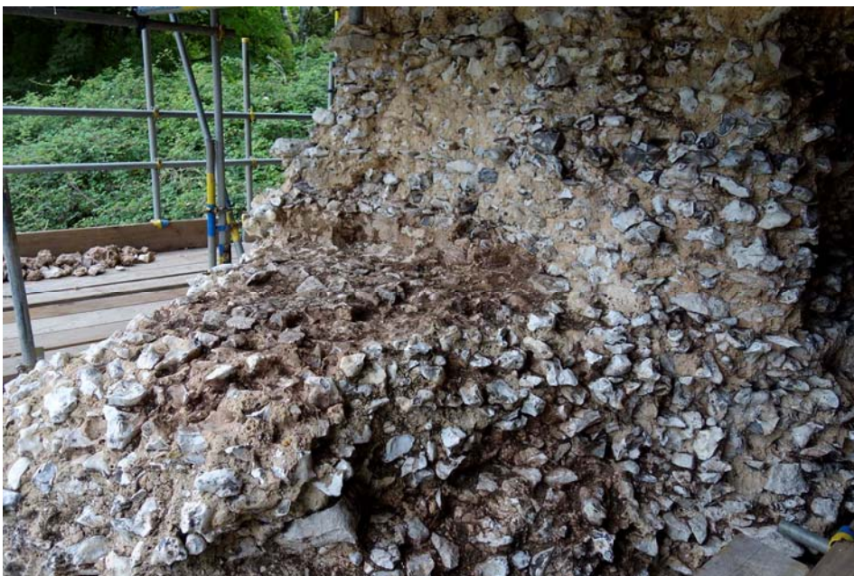
Figure 31. Remains of stair vice in the west wall of the gatehouse, leading from first to second floor level. The flat area (centre of photo) stained by earth is identified as the bottom of the vice.
