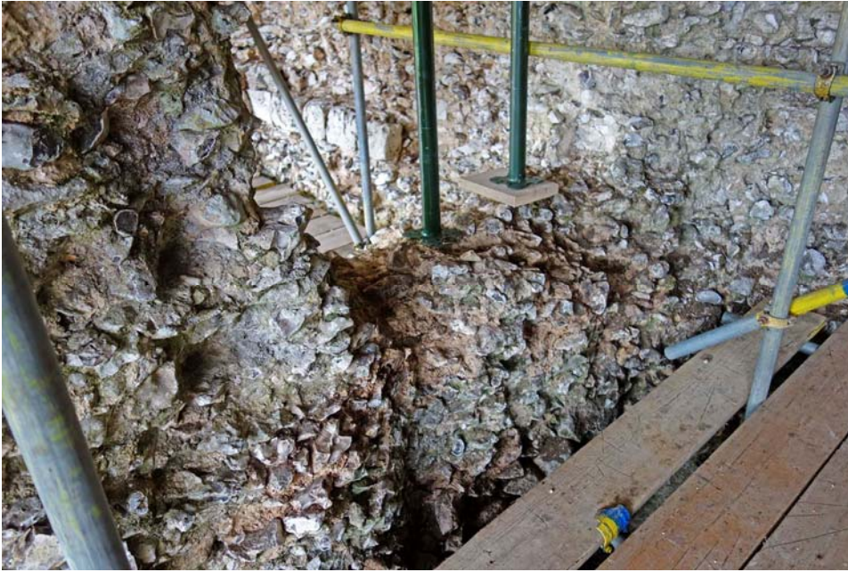
Figure 22. View WNW at corework of step through the spine wall at first-floor level. The line of chalk blocks in the north wall, visible through the doorway, defines the higher first floor level over the gate passage.
