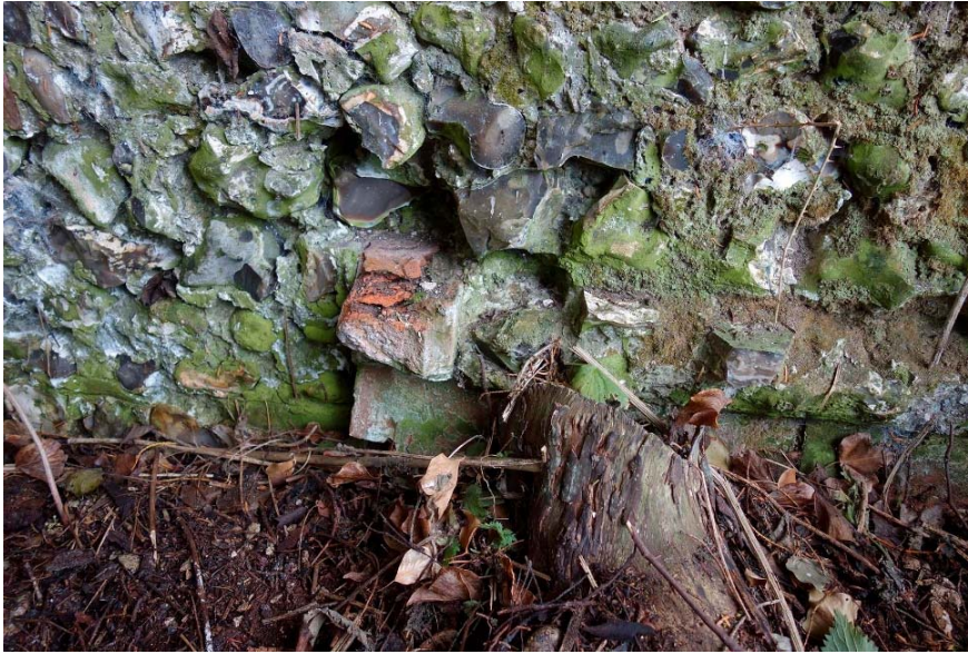
Figure 37. Brick embedded in flintwork of abutting north wall of the square additional building.
