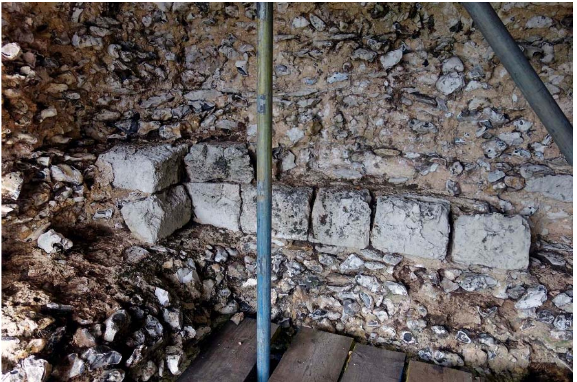
Figure 17. Row of chalk blocks on inner face of north wall of gatehouse, above the entrance doorway, here identified as deriving from the first floor over the gate passage.
