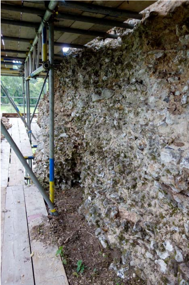
Figure 9. East face of gatehouse, oblique view south, showing possible springing of curtain wall (behind scaffolding standard).
