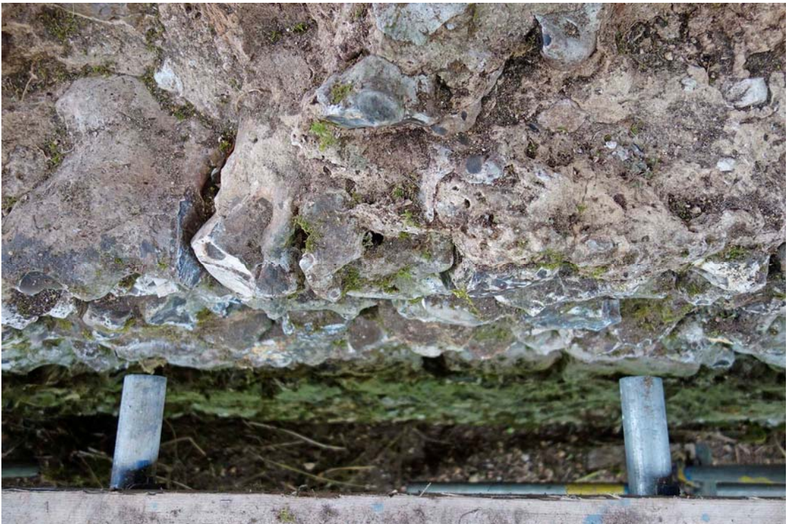
Figure 10. Possible original external wall face: the lowest 4m of north external wall, towards the NE corner of the gatehouse. Above this level (top half of photo) the facing has slumped away.
