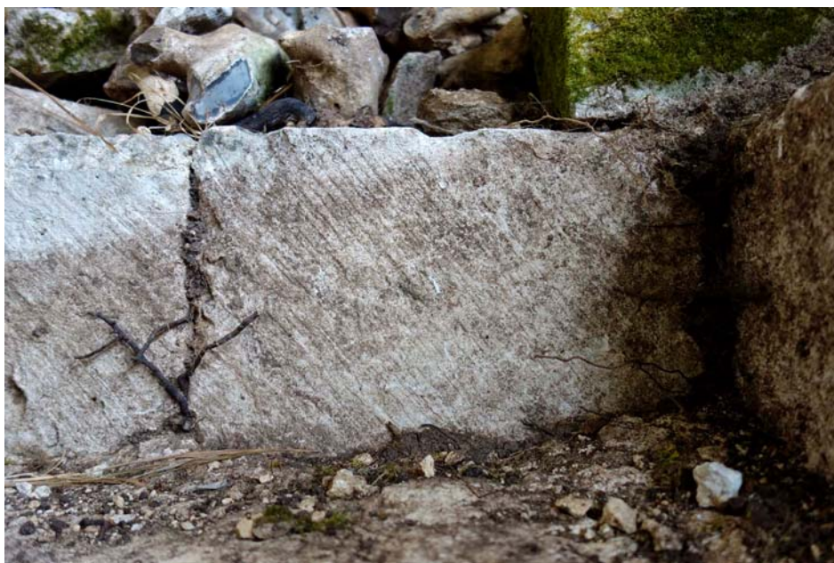
Figure 35. Tooling of masonry at rear of niche.
