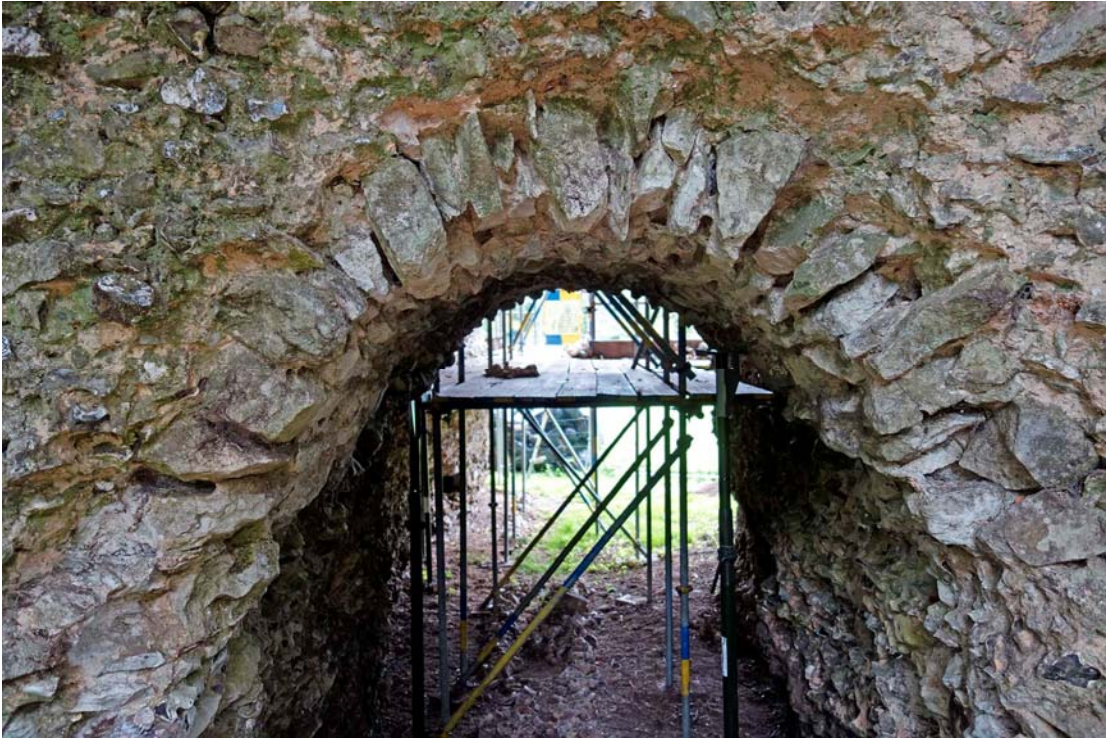
Figure 12. Entrance arch seen in section, showing voussoirs.
